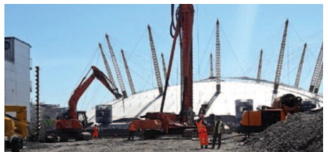
CFA piling with the powerful Llamada P160TT
