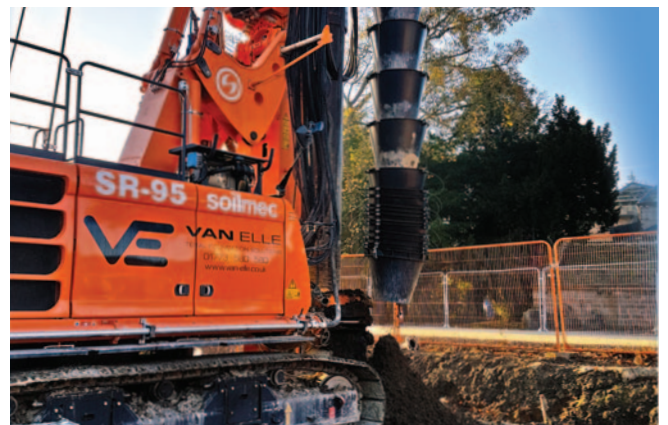
Cased CFA piling at Grantley Hall hotel and leisure
