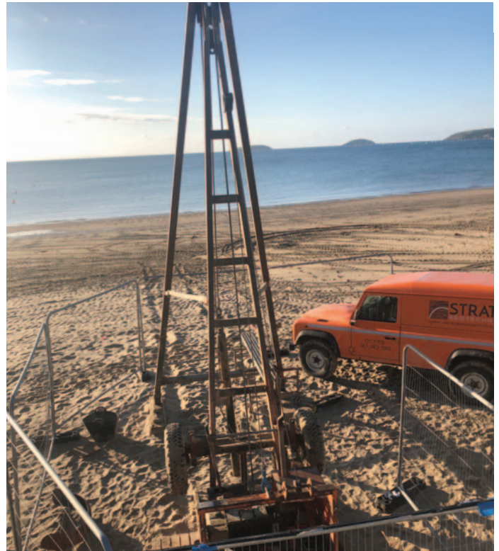
Cable Percussion sampling for the re-development of a UK holiday park.
