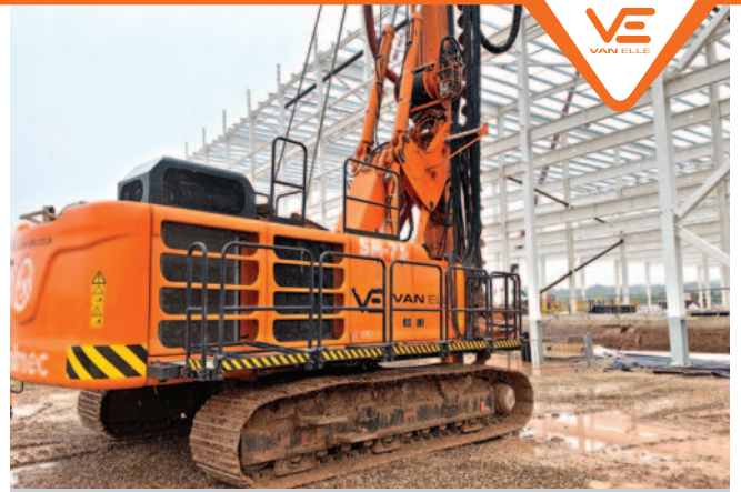
Solimec SR-75 providing foundations for large warehouse development in Mansfield
