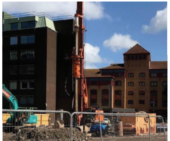
Coring works in Bristol for BAM Construction.
