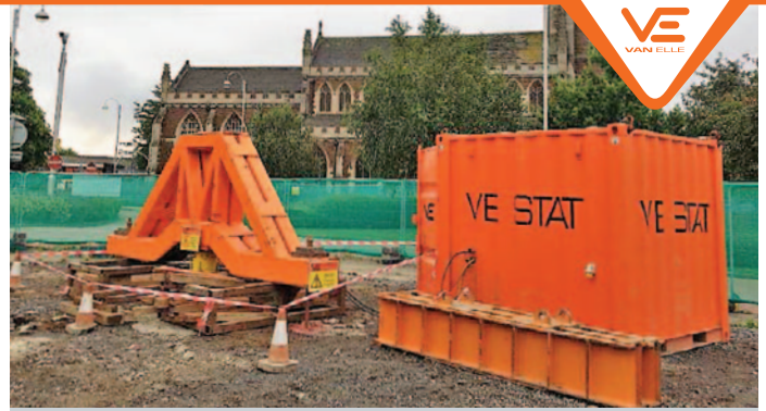
Load testing for pile bearings by STRATA Geotechnics
