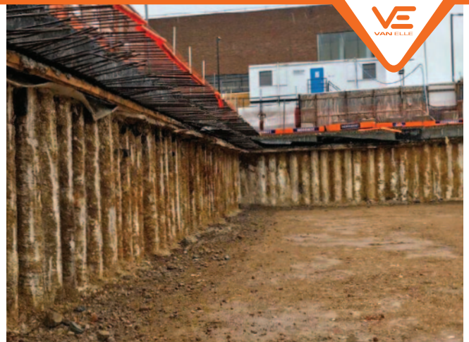
Retaining wall installation in St Albans, London for basement scheme
