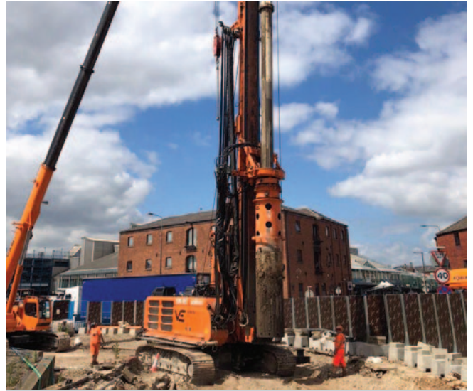
Large diameter rotary piling for A63 improvement scheme
