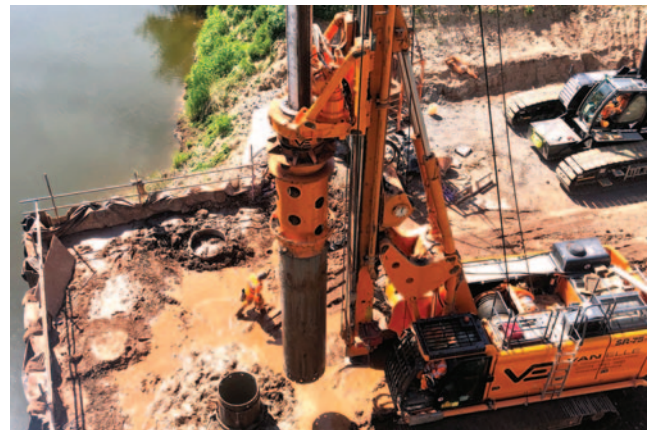
Large diameter piling for A4440
