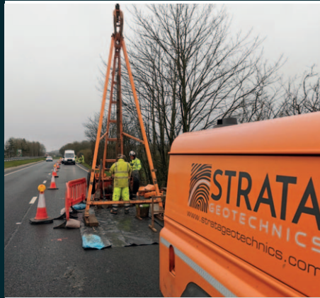
Cable Percussion Drilling
