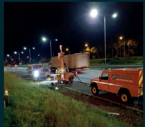
Drilling on Highways
